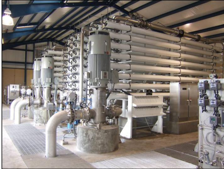
Figure 5 – Membrane Feed Pumps and LPRO Units
