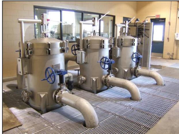
Figure 3 – Membrane Feedwater Cartridge Filters
