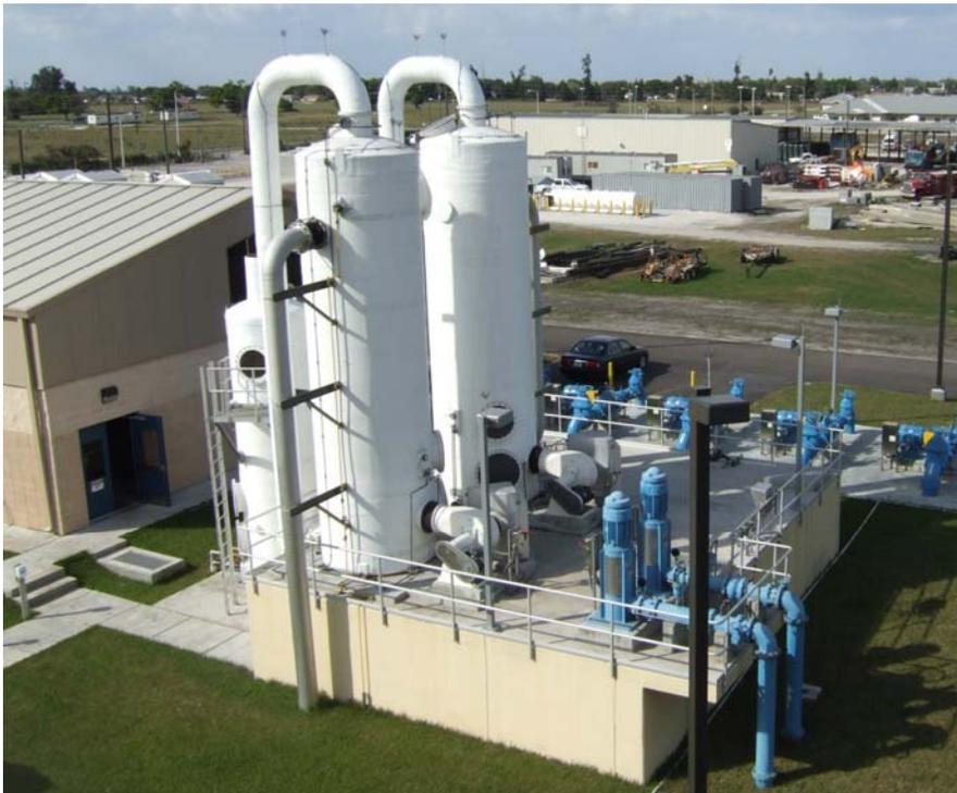
Figure 6 – Degasifiers, Clearwell, and Transfer Pumps
