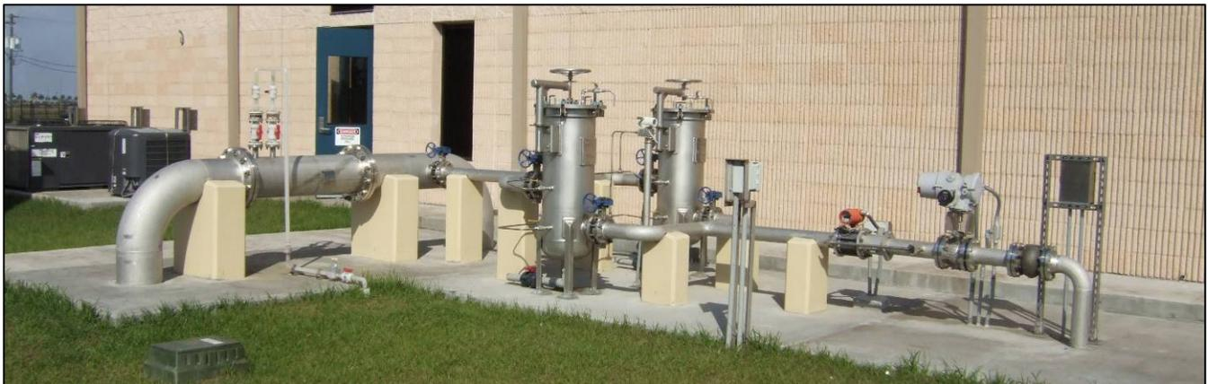
Figure 4 – Acid Injection Point, Bypass Cartridge Filters and Control Valve
