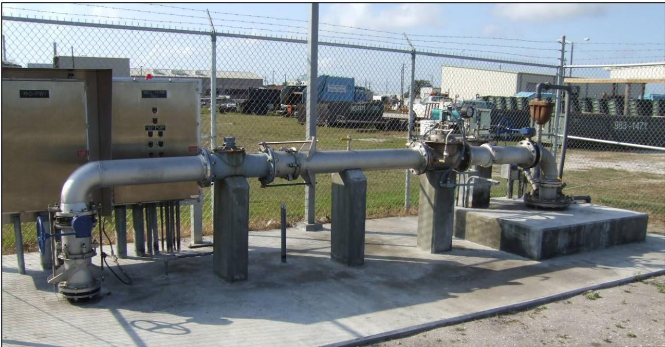
Figure 2 – Well PW 1, Typical Floridan Aquifer Production Well
