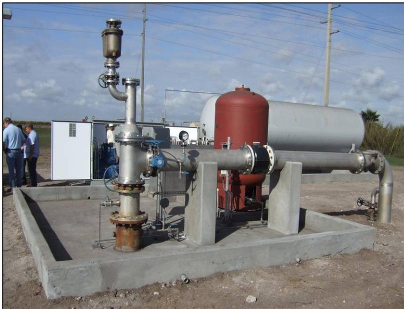
Figure 7 – Concentrate Disposal Deep Injection Well
